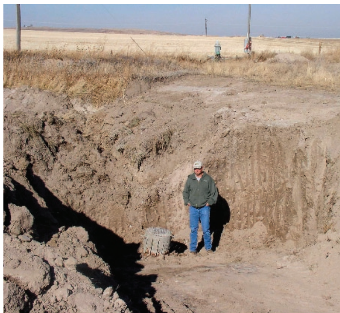
Dan Strickler, Minidoka County SWCD, stands in a well that is to be capped. When these wells were functioning, they produced a loud suction noise as runoff contaminated with nitrates, pesticides, bacteria and sediment rushed down into the aquifer.
